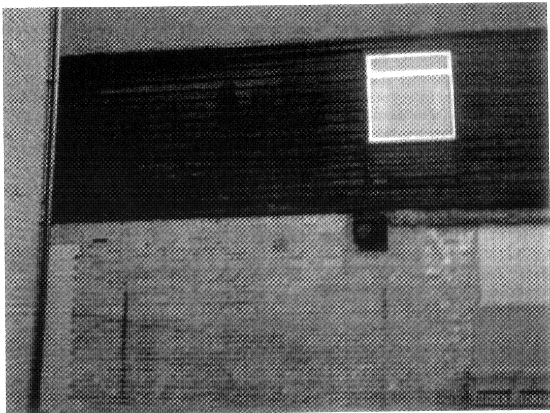
One of the Club overlooking windows, grills and fan opening
